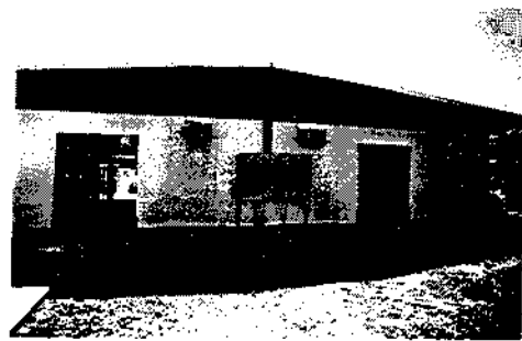
Figure 2b. Grower Facility
